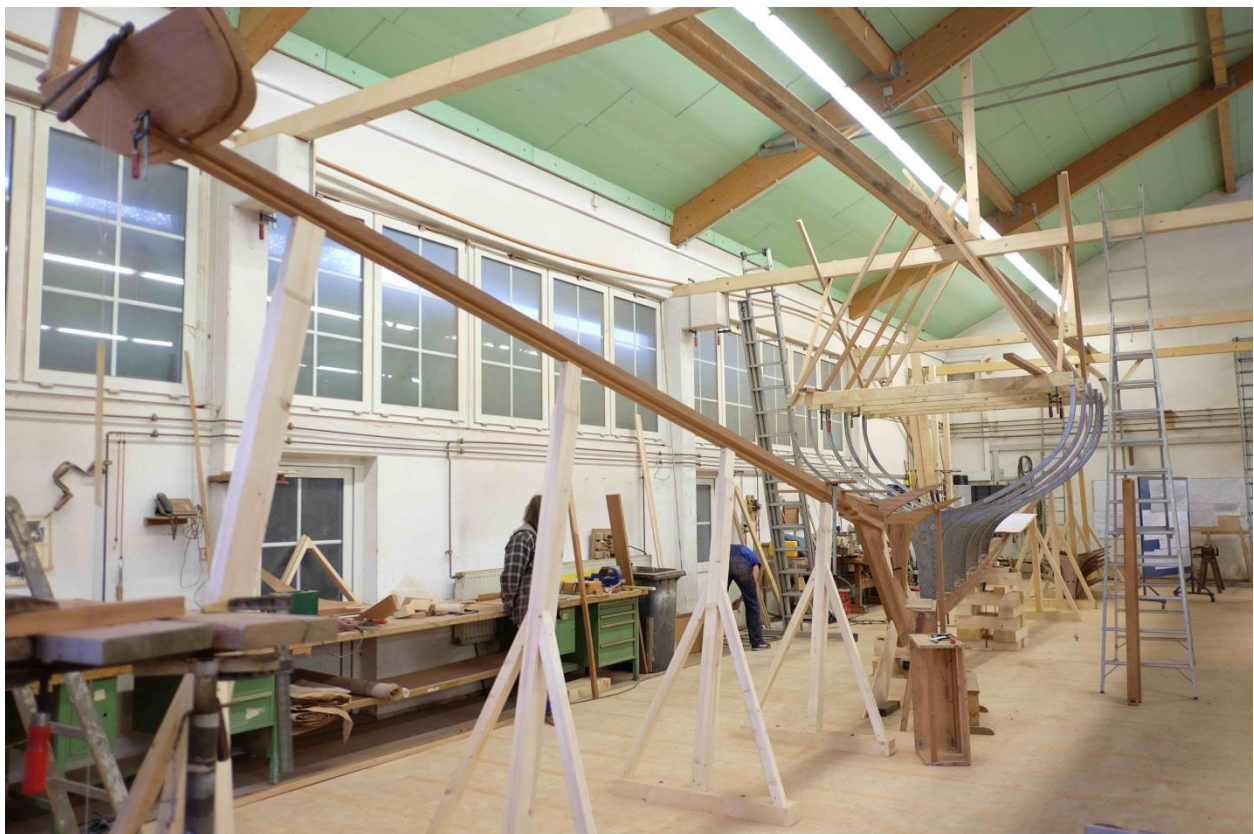
October 2015 – start of the construction Photo: Juliane Hempel. All rights reserved.
